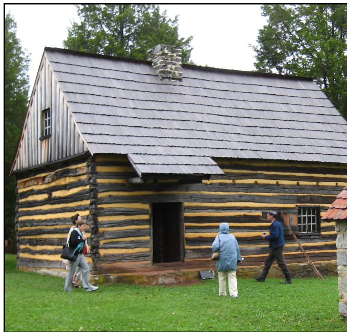
The Bertolet cabin at the Daniel Boone homestead is a typical log home built by early German settlers.
